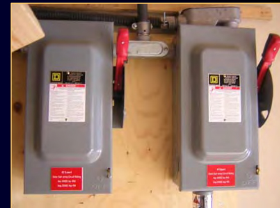
DC array switches
