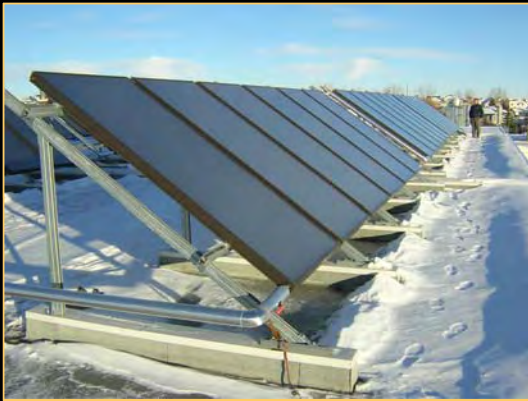
Okotoks swimming pool solar heating
