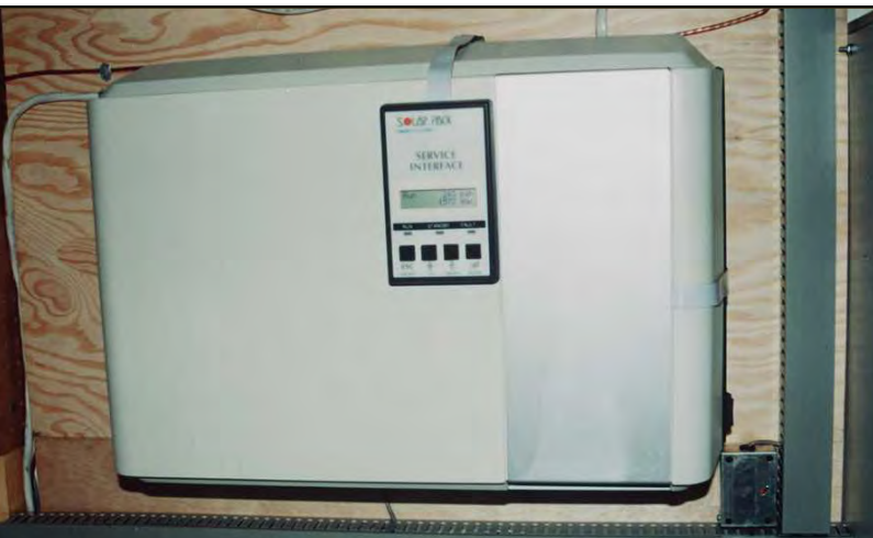
2 kW ARISE GX 5000 inverter.
