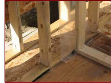
Double-stud 2x4 walls with U si -0.10 (R-56) cellulibre
