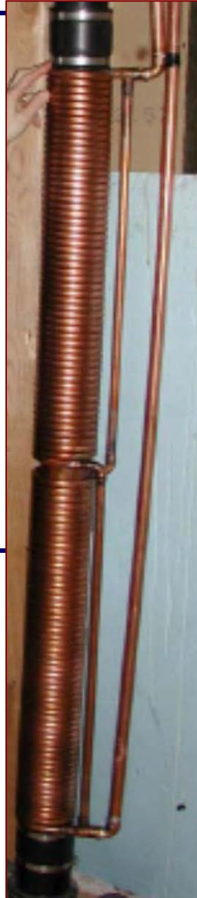
Drain water heat recovery
