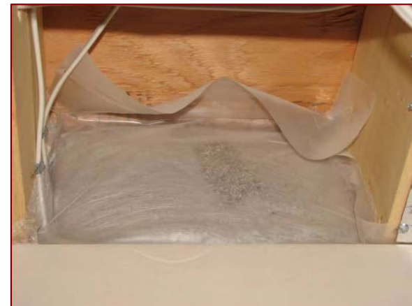
Rim joist vapour barrier
