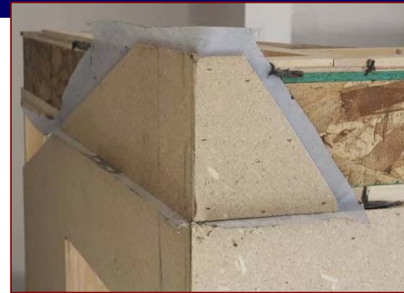
Rim joist air barrier wrap
