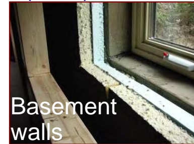
Double-stud 2x4 walls with U si -0.10 (R-56) cellulibre
