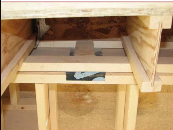
Spreader plate joints sealed
