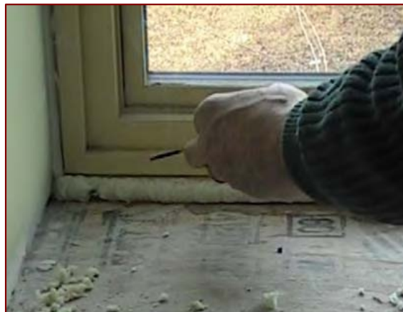
Windows foamed All penetrations sealed
