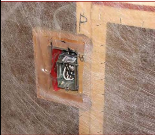
Electrical poly-vapour hats and backers
