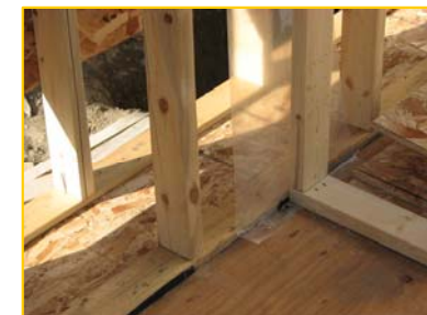
Double-stud 2x4 walls with R-56 cellulose
