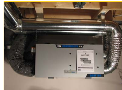
Heat recovery ventilator 80% efficient
