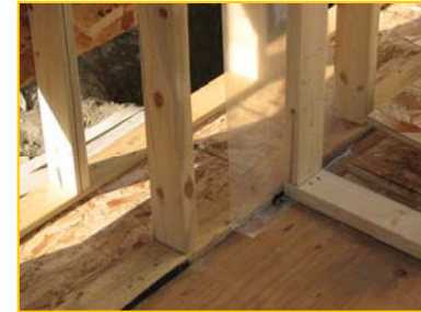
Double-stud 2x4 walls with R-56 cellulose
